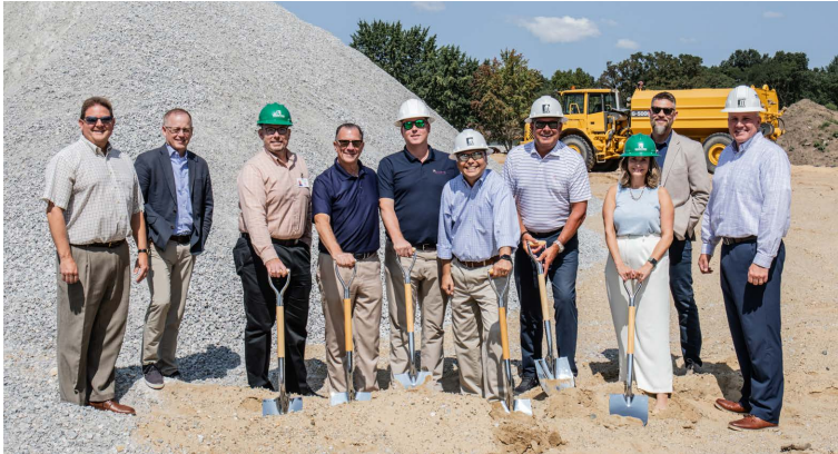
Geerlings Development and KJK developers broke ground on the Lakewood Place Apartment Village project.
